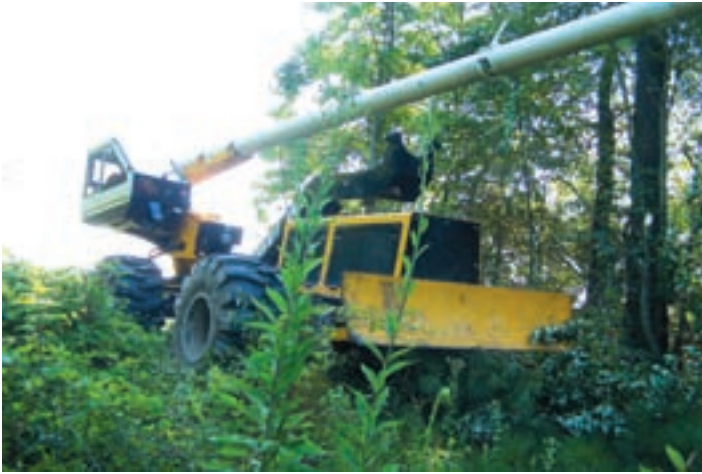
Wolf Tree owns nine Jarraff All-Terrain Tree Trimmers in addition to five other mechanical trimmers.
