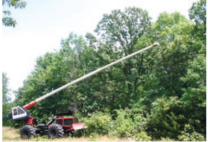
The bucket trucks Hentges used at the beginning of this job were not tall enough to reach the top branches. Jarraff All-Terrain Tree Trimmers were brought in to compliment the bucket crews.
