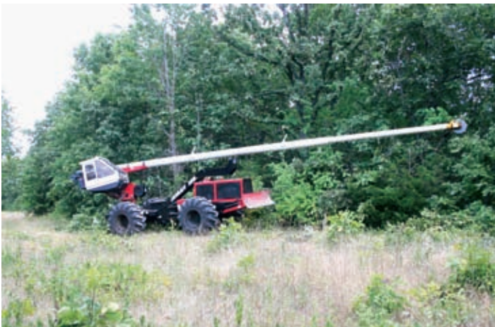
All-terrain tree trimmers make ROW maintenance safer by reducing the need to have climbing crews cutting above the lines. The Jarraffs allow operators to stay safe and comfortable in the cab while trimming.
